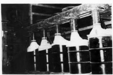
DRUMMING of yellow cake requires little attention. Wet pellets are formed by extruding concentrate filter cake through a screen; pellets travel on steel conveyor through Proctor Schwartz drier. Dried pellets are screw conveyed to drums.
